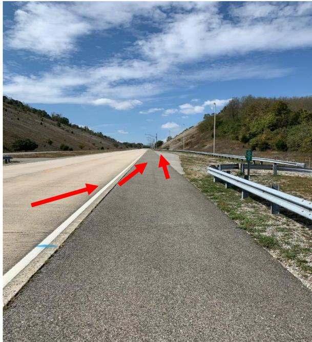
Figure 2. Extended shoulder for lane deviation.
